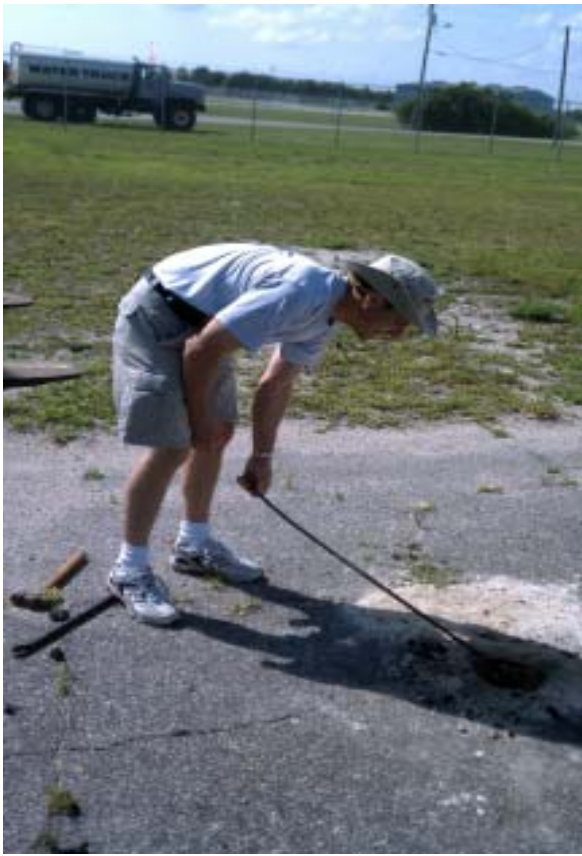
Paul on tie down relocation duty.
